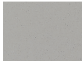
A31 New Concrete
